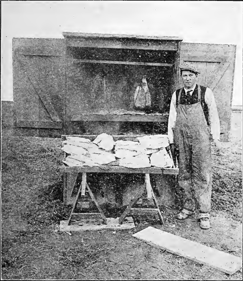
FIG. 3.—The smokehouse in operation. Some of the fish are on trays, one of which has been removed for the purpose of photographing. Others, in wire slings, are suspended from rods near the top of the house.
